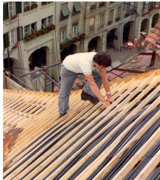
Figure 7-4 Roof collector below tiles installed between rafters, 1978 [Grimm 2007]
