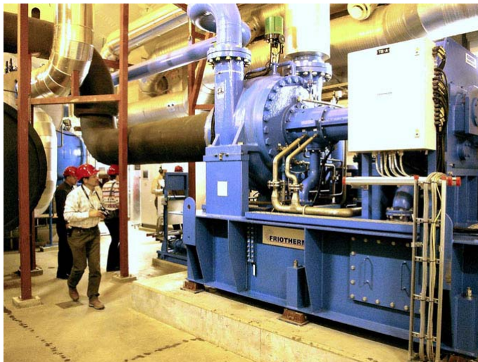
Figure 8-11 18.4 MW heat pump of the Viken Fjernvarme of the district heating system of Oslo [Friotherm 2008]
