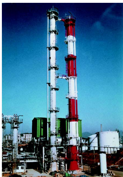
Figure 7-18 One of the first distillation plants with vapour recompression [Sulzer Chemtech, CH-8404 Winterthur]
