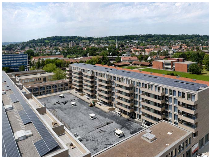
Figure 8-9 Eulachhof, Winterthur. Photovoltaic panels to drive the heat pumps and aeration. [Allreal, CH-8050 Zürich]
