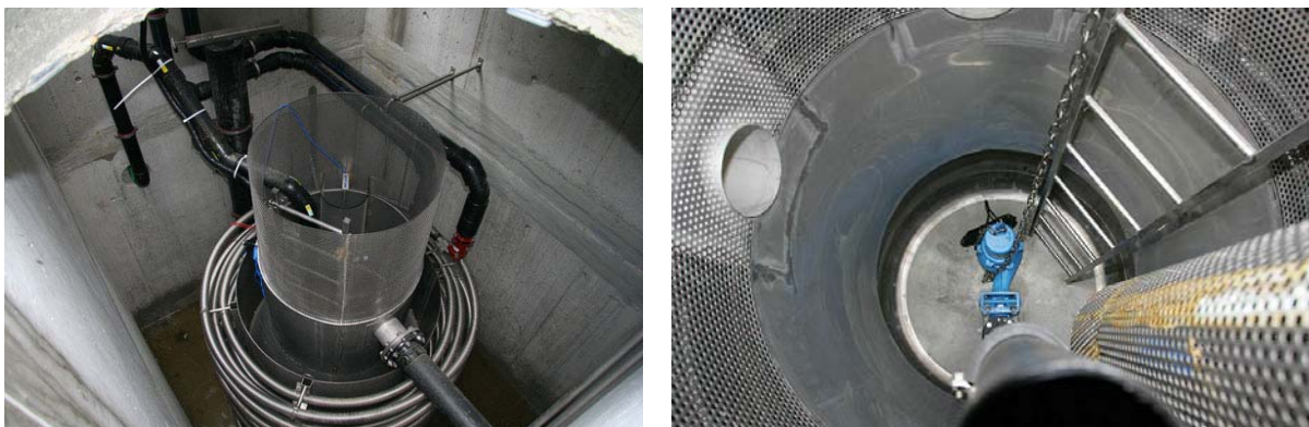
Figure 7-15 Latest version (2007) of the FEKA tank for the heat recovery from raw domestic sewage. Left: heat exchanger tubes, right: solid separation zone. Photos Eulachhof Winterthur [Kalberer 2007]
