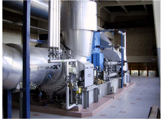
Figure 5-32 New radial compressor for the evaporation crystallisation at Aarberg, 1991 [Zuckerfabrik, CH-3270 Aarberg]
