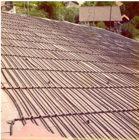
Figure 7-3 Roof collector with polyethylene tubing on the roof, 1978 [Grimm 2007]
