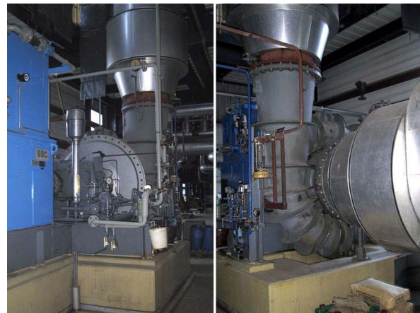
Figure 5-30 Second radial compressor for the sugar solution concentration at Aarberg, 1984 [Zuckerfabrik, CH-3270 Aarberg]
