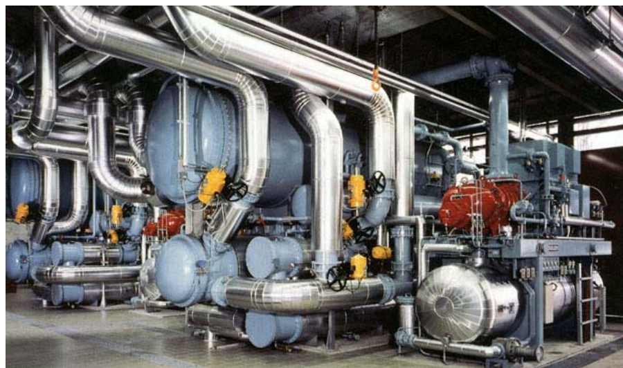
Figure 7-13 3.9 MW ammonia heat pumps at EPFL, 1986 [Friothersm 2008]
