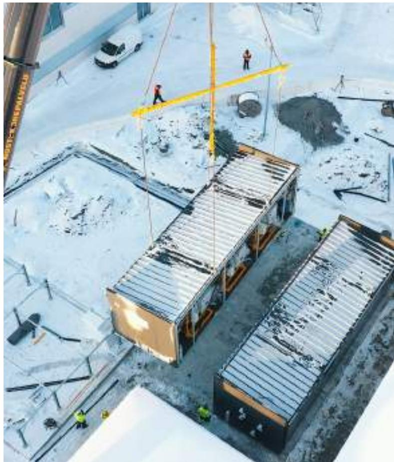
Factory-installed and factory tested heat pump plant modules being delivered to the site.
