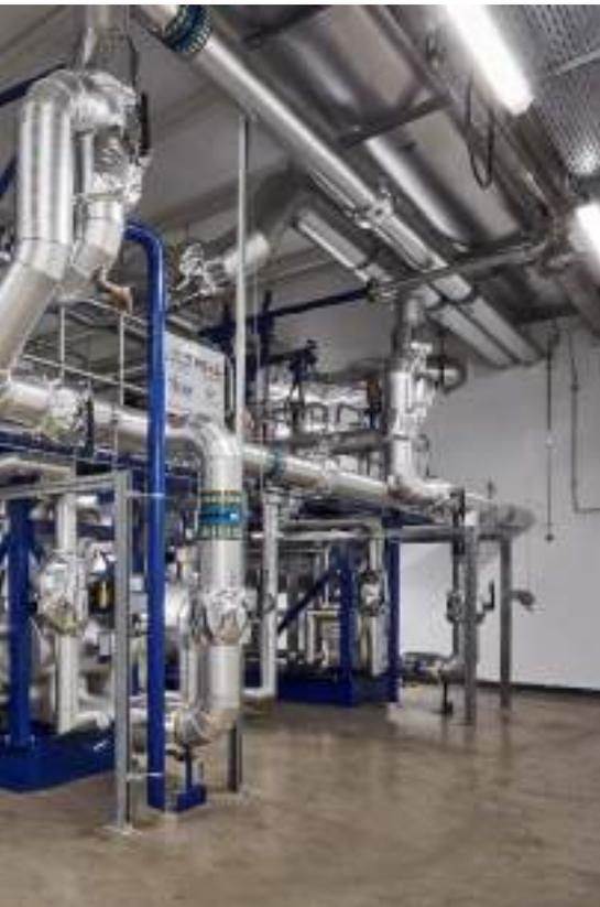
The two 2.65MW water source heat pumps installed at Queens Quay are the primary heat generating technology on the development and also make it the largest project of its type in the UK.
