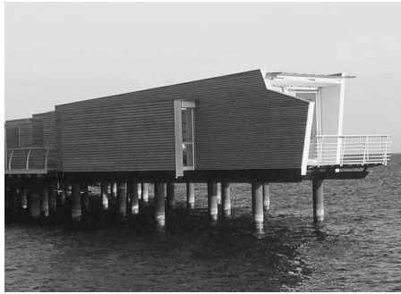
Figure: Hotel Palafitte with heat pump
