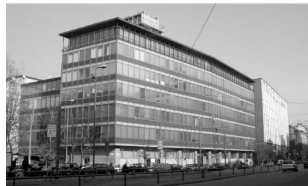
Province of Milan building, equipped with a ground-source heat pump
