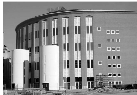
University of Bocconi, equipped with a ground-source heat pump
