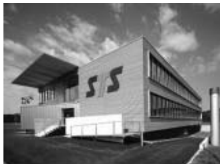
Figure 3 Swiss commercial building, heated and cooled with a heat pump.
