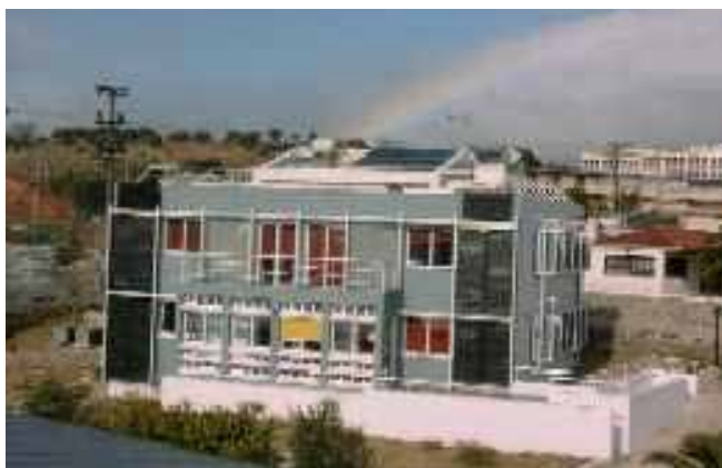
Figure 6: Office building of Centre for Renewable Energy Sources (CRES).
