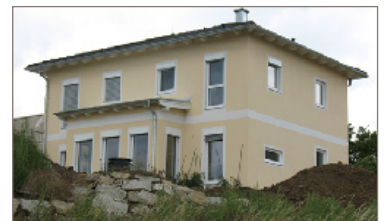
Type: one-family house Heated area: 130m 2 Location: Austria Heat pump: ground source; vertical drilling Measured SPF: 4
