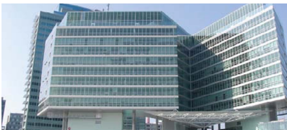
Type: administration building Heated area: 28.000m 2 Location: Austria Heat pump: ground-source (energy piles)
