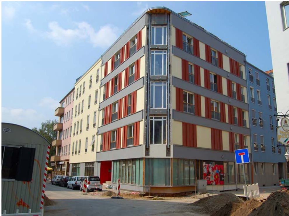
Photo 2: Building after renovation
