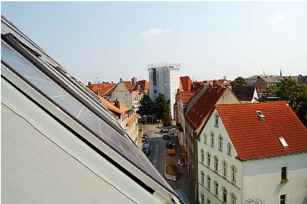
Photo 4: On-site photovoltaic system
