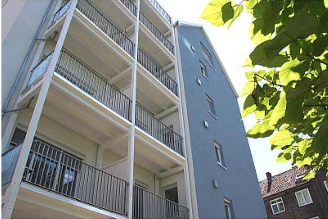
Photo 5: House front with air outlets of decentralized ventilation units
